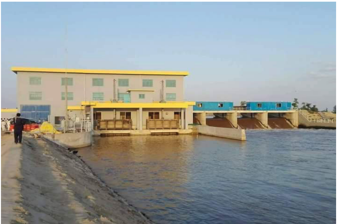
Figure 2. A view of completed Pakpattan hydropower project.
