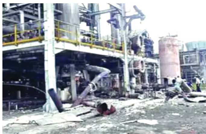
Figure 5. A major explosion ripped through an ammonia-urea factory in the Namrup-2 unit.
