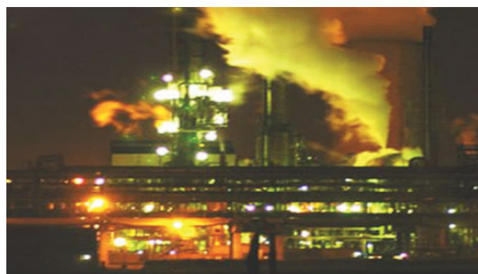
Figure 2. Fire and explosion due to a mixture of hydrogen, nitrogen and ammonia at the Terra Nitrogen Plant, UK.
