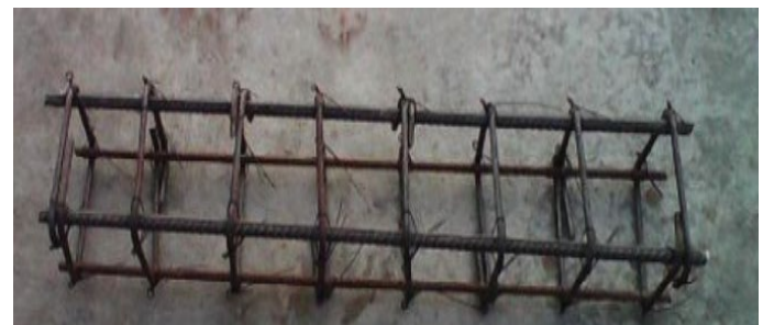
Figure 4. Reinforcement details of short column.
