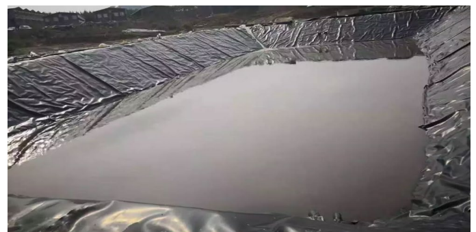
Figure 1. Illustrates the anaerobic treatment process employed for the treatment of pig wastewater in a lagoon.
