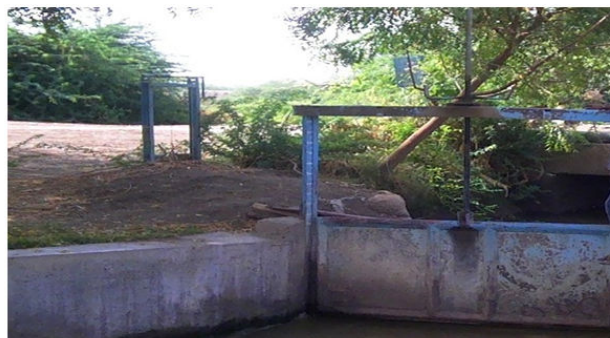
Figure 2: Head and cross regulators of typical monitored secondary canal-1 of primary canal-1.
