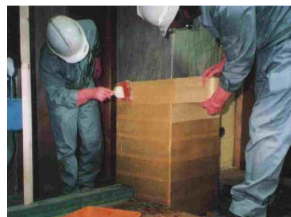
Figure 14: Attachment of Kevlar Mat with Epoxy [25,33].
