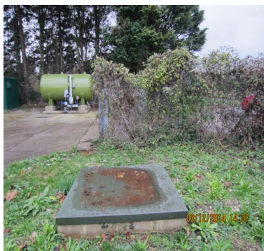
Figure 1: At the Lord of the Manor site, the existing below ground surge vessel, which can be seen in the foreground, was abandoned and the new tank installed in a location nearer to the water main.
