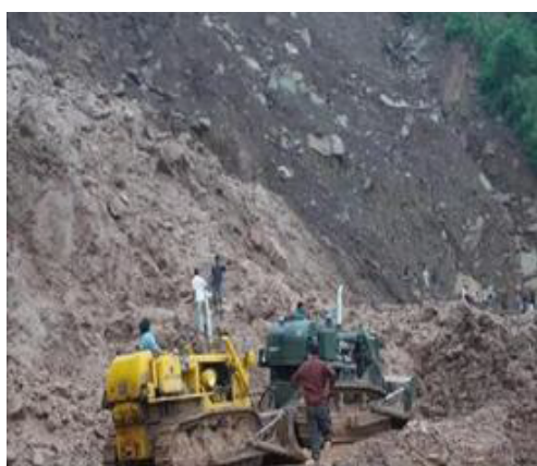
Figure 9: Clearance of debris from the road.
