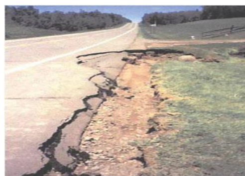
Figure 10: Deteriorated drainage system.
