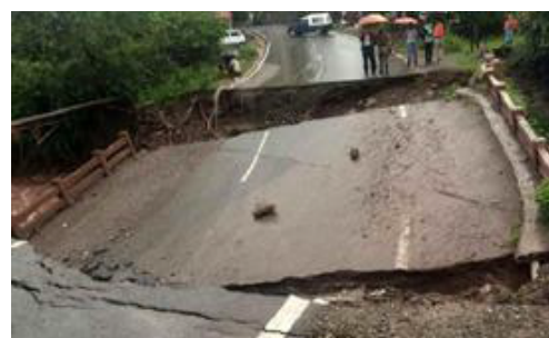
Figure 2: Road cracking because of floods.
