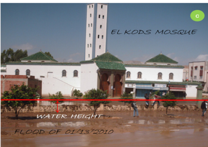
Figure 4. Al Massira market after the flood of 13/01/2010. El Kods mosque after the flood of 13/01/2010.
