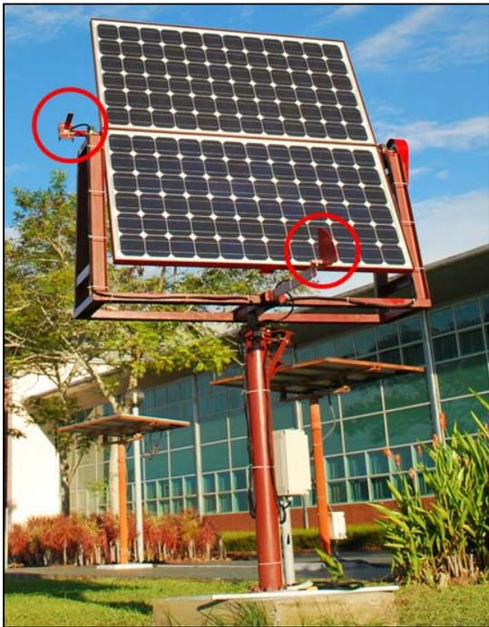
Fig. 14: Placement of the sensors on the structure
