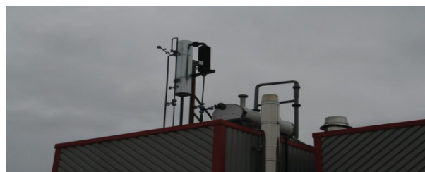
Figure 2: A picture of a permanently installed LERK. Picture courtesy of Global Heat Transfer.
