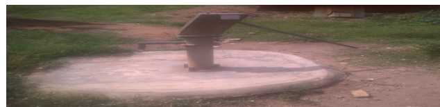
Figure 3: Non-functional hand pump borehole, a World Bank assisted project at Oke-meji community, Ward 11 Akure South L.G.A.
