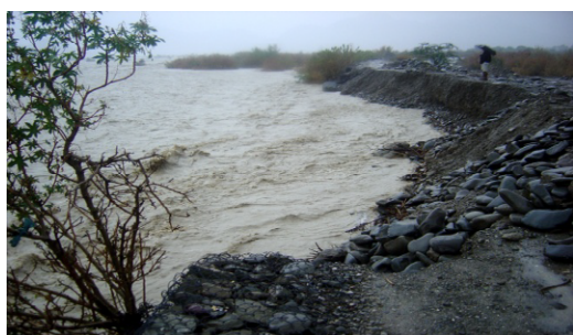
Figure 3: River Kajo Overtopped levee at District Ghasrghand during flash flood 2013.
