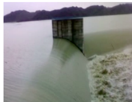
Figure 2: Spillway of the Pishin Dam with bankfull flow during flash flood in the stem of Sarbaz River.
