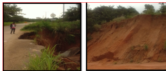
Figure 2: Image showing the erosive effects on the Okigwe-Isikwuato road and the sloped gully walls.
