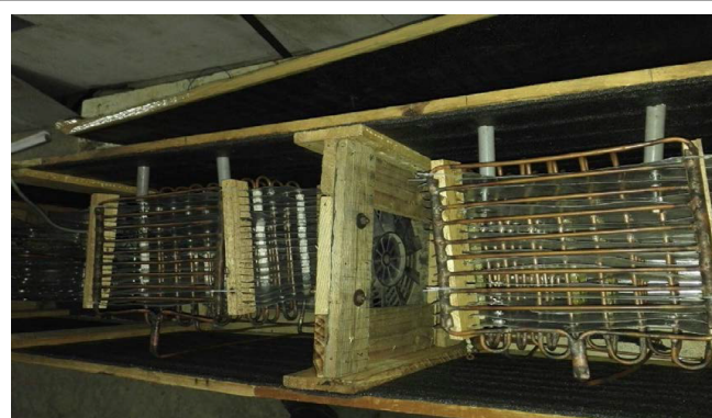
Figure 11: Falling film desiccant air conditioning system.
