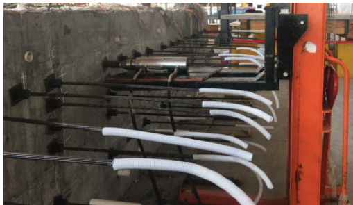
Figure 5: Prestressing the steel strands.
