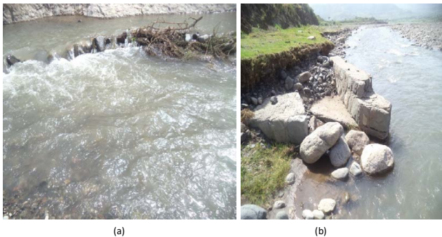
Figure 11. Traditional diversion structure and current condition of the designed intake structure.
