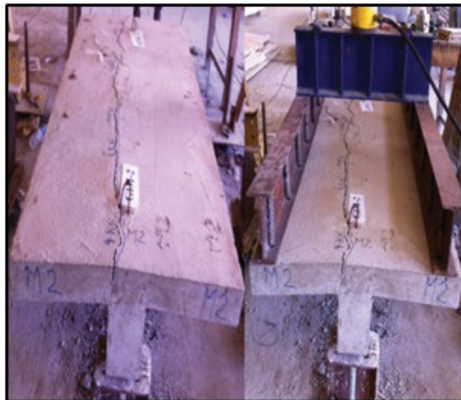
Figure 7. Cracks pattern of specimen GIM-2.
