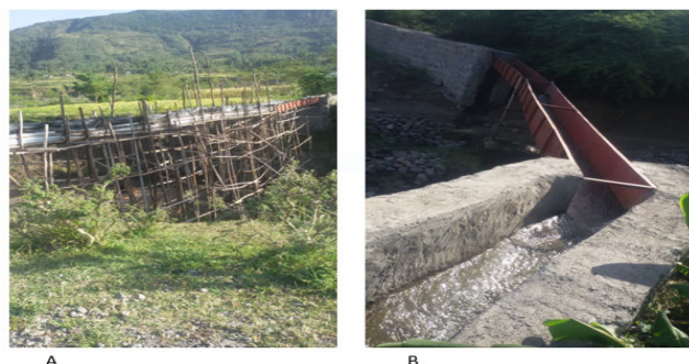
Figure 6. Malfunction of waterway transmission bridges of SSI scheme: Water Way Bridge at Gebrie amba SSI (A), Water Way Bridge at Jarssa SSI (B).
