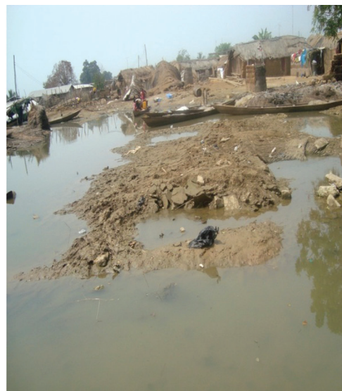
Plate 2: Collapsed mud houses.
