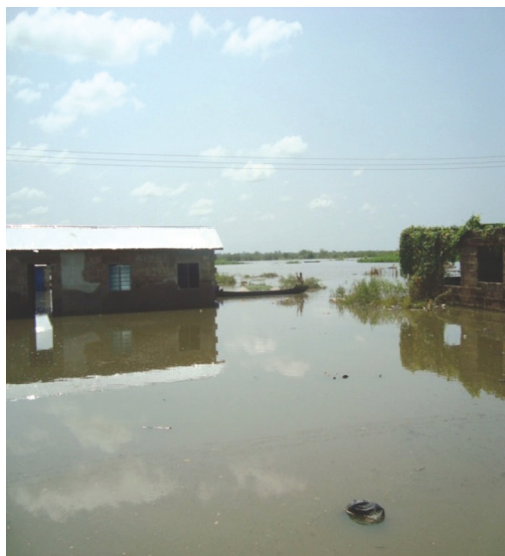
Plate 1: Block house that had been able to resist flood.
