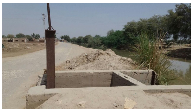
Figure 6: Non-modular irrigation outlet.
