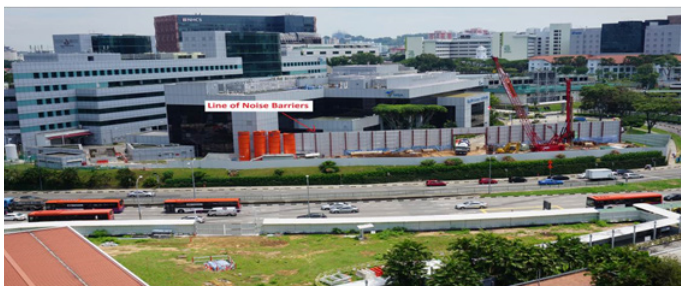
Figure 2. Noise barriers installed in front of existing building.
