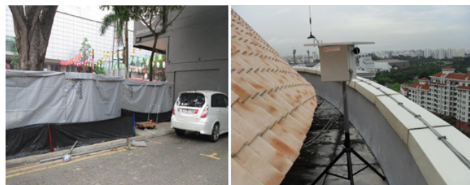
Figure 3. Noise blanket in public car park (left) and noise meter on the roof top (right).
