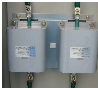
Figure 13. Noise filters for grounding system [31].
